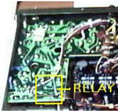
FINAL unit relay
